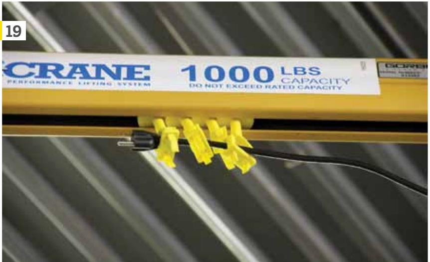
With our Shop Crane installation almost completely finished we installed a tagline to hold the hoists' electrical wires up off of the ground and ensure that they won't get tangled during use. The wire was threaded through the yellow tagline clips along the bridge. These will space out as the hoist is moved after the wire is plugged into an extension cord.
