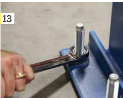
Next, we went ahead and tightened the nuts to the anchors at the base of our columns, so that each side of the structure was stiff and secure for the installation of the bridges. Remember to check and retighten the bolts a few weeks after installation. You might choose to cut the anchors after tightening so that they are flush with the bolts, to avoid the risk of tripping over the tall bolts.
