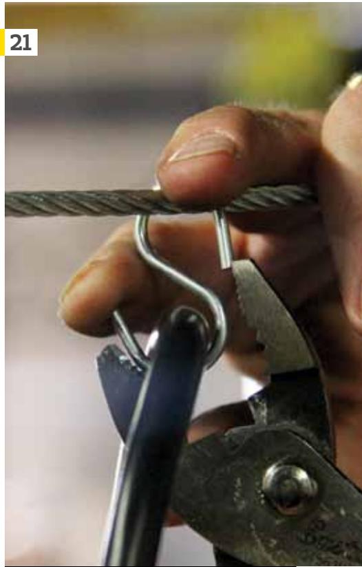
S-hooks were hung on the cable and tightened around the extension cord so that they can move freely as the bridges are moved from front to back.
