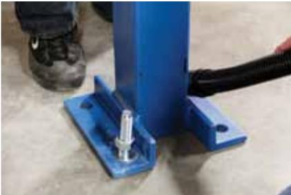
Using a hammer, Fisher drove the anchors into the holes before applying the bolts, without tightening them. We needed to be sure there was play in the column so that the rest of our installation would go smoothly.
